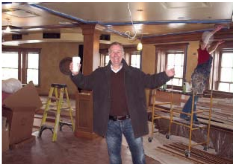
General Contractor, Maurice McNally, on the job!
